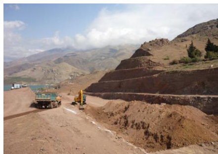
Figure 2. A view of the cutting slope with four berms of 4 m width and 6 m height (1H: 2V) and heavy works during the 5-6 m excavation on the toe of slope along 41+400 to 42+200 km of Qazvin-Rasht freeway
