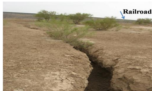
Figure 2. Vertical crack near the railroad in Semnan plain
