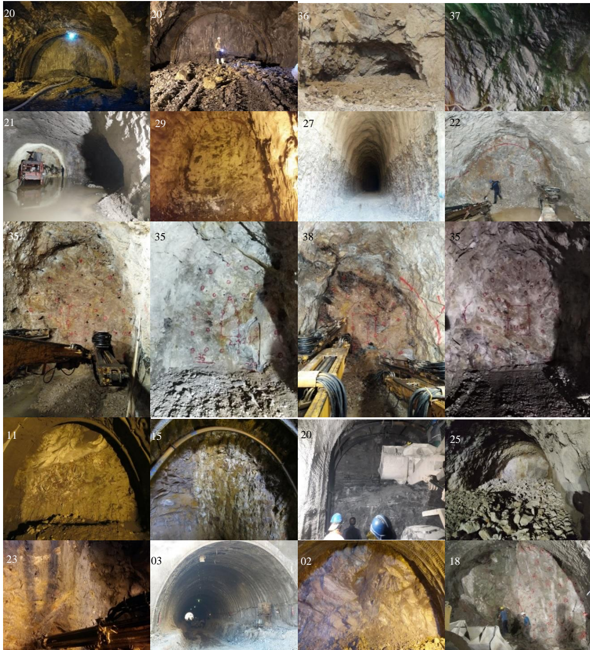
Fig. 2. Images of some of the studied tunnels (the number of each image corresponds to the tunnel number in Table 1).
