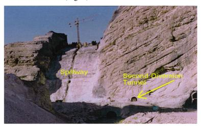
Fig.5. A photo of the second diversion tunnel in the left abutment.
